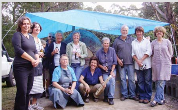
Above: Pizza Oven building bee in April and the builders at the end of the day with Dee squatting centre front.
